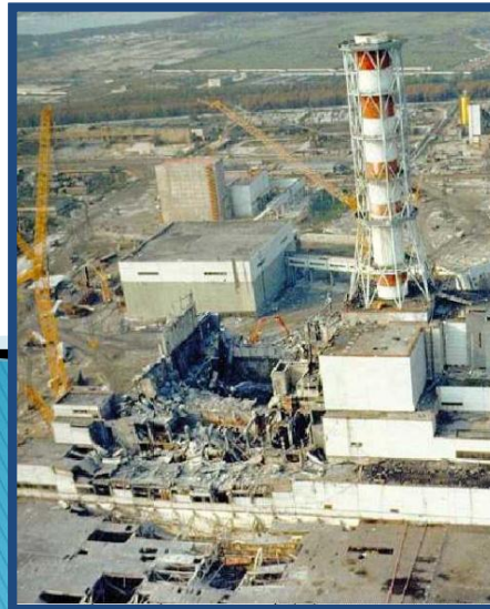
Tchernobyl Reactor Building damage
